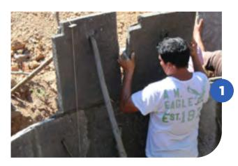
We follow the same way to put the second row of plates for the wall into place, using the chosen propping system. The plates of the upper wall are stuck overlapping the joints on the first row of plates to complete the whole wall.
