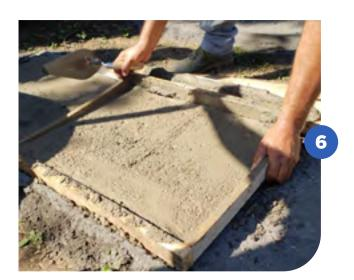
Wait a few minutes to take off the mould holding the corners diagonally so the shape of the plate is not altered.
