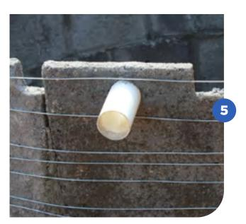
On this row we put the plate with the hole for the water escape. We put it in a convenient place, where there's the possibility of taking advantage of the overflow to irrigation and so it doesn't flood the front of the house. This hole must be covered with a netting to prevent the entry of little animals, dirt and dust.
