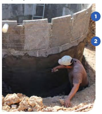
Brush the walls to remove the loose sand and apply two thick layers, plastering until covering the whole wall. It is important all the turns of the wire are covered.
