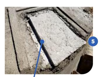
Around the plate where the door will be installed we make a frame to avoid the water from flowing into the cistern directly. This will protect the cistern from earth and will facilitate the installation of the door.
