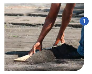
Make a layer of fine sand leveled to the ground where the plates will be manufactured.
