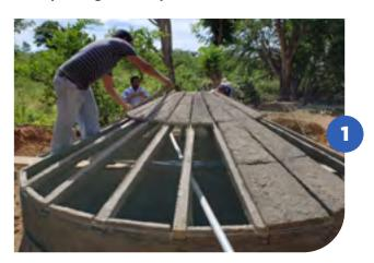
After the assembly of the beams with one of the two systems of central pillars we put the roof plates, one by one, leaning them on the beams with their smooth side facing in.
