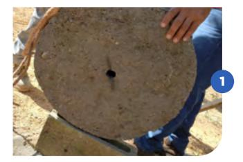
At the center of the cistern we apply some of the mixture in the form of a circle with a diameter of approximately 40 cm.
