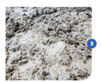
Finishing the plaster we make a mortar with water and cement (fifty-fifty) to brush the wall and the floor.
