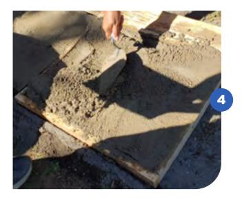
Distribute the concrete inside the mould giving special attention to the corners.
