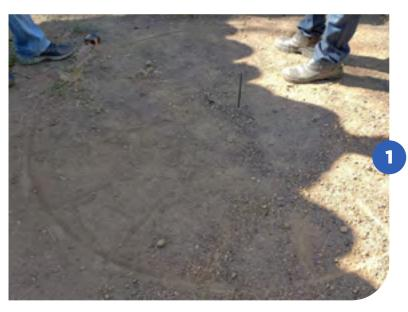
In an open and clean space, different from the cistern's site, we mark on the floor a circle of 1.75 m radius that equals 3.5 m diameter. It's important the soil is very compact.
