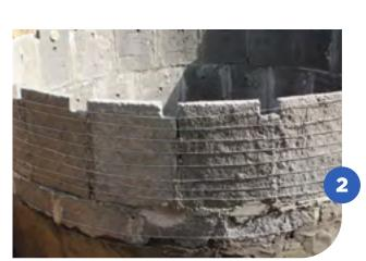
Each time a row is completed, we encircle all the circumference with number 12 galvanised steel wire. We repeat this procedure seven times. In other words, every row of plates will be encircled externally by seven turns of wire, as the pictures show. This wire works to strengthen the wall of the cistern.
