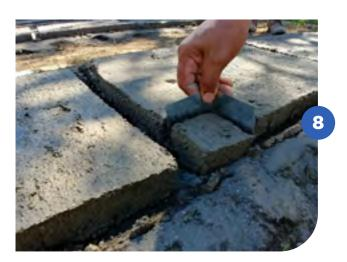
In 21 plates it is necessary to make a  $8 \times 8$  centimetre cut while the concrete is still fresh. This will be the upper row of plates, where the roof beams will be leaned over.
