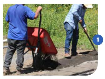
Like it was made with the plates, start making a layer of sand leveled to the ground where the beams will be manufactured.
