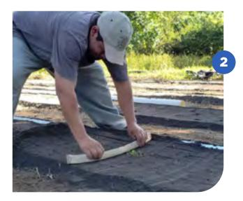
Drag the mould on the sand to make sure it take the round shape of the plate when filled with the concrete.
