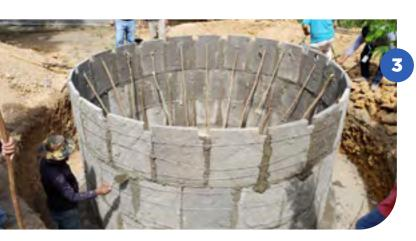
We put up the third row of plates for the wall in the same way we did the others, using a plumb bob and putting the joints perfectly together inside and outside. We do that paying attention to the lines and plates.
