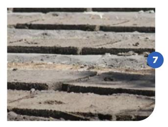
In all the plates, make a mark sinking a spoon near the edge as it can be seen here. This will make the suppporting easier when it's time to assemble the wall.
