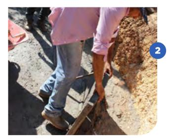
Put the mortar on the perimeter and stick the first plate. Continue the same way with the other plates following the round mark.
