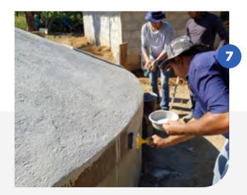
We paint the exterior of the plates cistern with lime or water-based paint. This refflects sunlight, reducing the temperature inside the cistern, protecting it from humidity and diminishing the possibility of future cracks and dilations.
