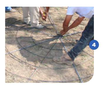
Then put the other 6 remaining iron bars in a way the structure has 16 radius formed by iron bars.
