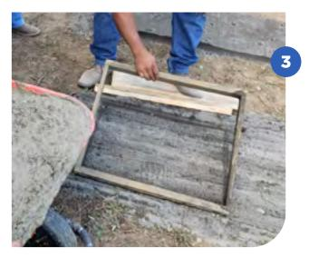
Lean the mould and fill it with the concrete.
