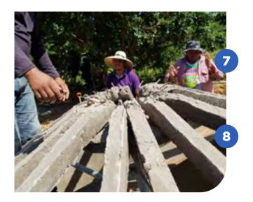
Each beam's iron hook is placed facing up, side by side, forming a little circle at the cement cover.
