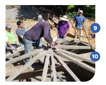
After all the beams are in their places we encircle the hooks with many turns of wire.
