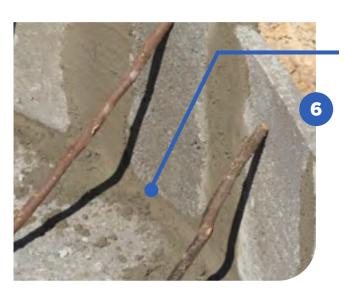
With the mortar we make a kind of excess border on both sides of the plates next to the ground so they fix well on the base.
