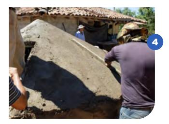
We complete the plaster of the entire cistern with the same material of the external wall.
