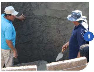
With the mixture we plaster the interior covering the entire wall. Smooth it to have a good finish. This plaster must not be too thin. It's important to pay attention if the entire wall is plastered and there are not any cracks.
