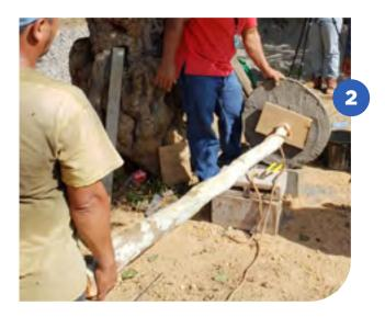
Upon this mixture we fix the central pillar with the end with the two pieces of wood facing up.
