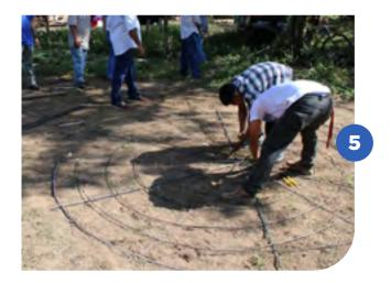
Put the other 8 mm iron bars in a concentric way with a distance of approximately 55 cm from the main circle tying the ends with wire.
