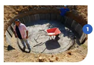
Once we choose the propping system, we prepare the mortar to assemble the plates and carefully transfer them to the interior of the well. We can lean them on the walls.
