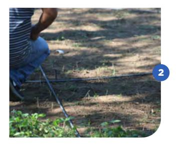
Use the 8 mm iron bar of 6 m in length to form the circle that was marked, tying the iron ends with wire and a stake.
