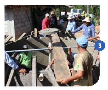
We fix the pillar with four wires crossed perpendicularly. We also could fix them with two pieces of wood, propped and tied.
