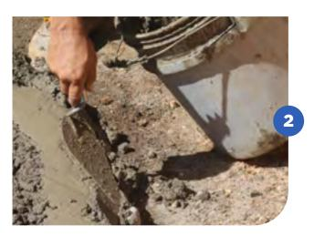
Fill approximately one half of the mould with concrete.
