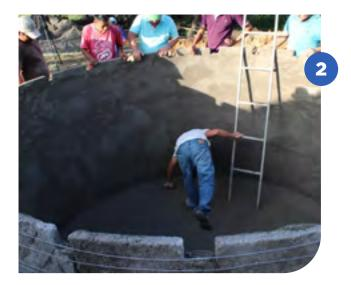
On the floor of the cistern we mix the mass and the diluted waterproofing.
